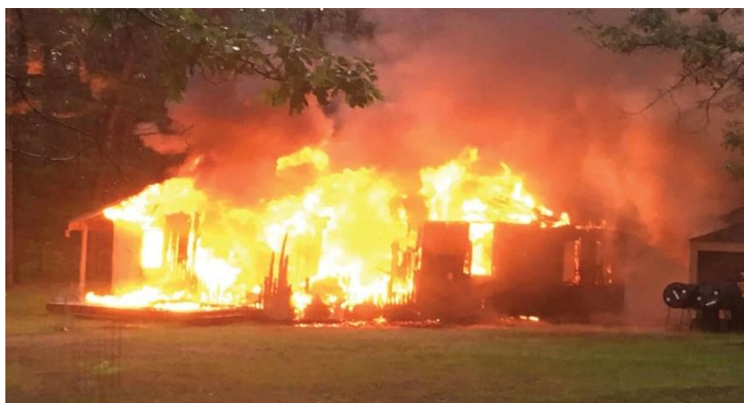
Figure 8 (b) A snapshot of a house gutted by an electrical fault down to ashes.
