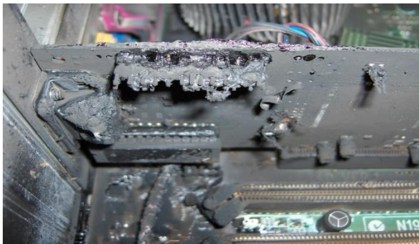
Figure 8 (a) Snapshot of the electronic circuit of a computer damaged due to electrical surge triggered by lightning.
